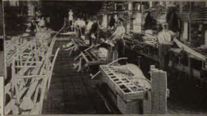
Manufacturing plows at the Avery Works, Louisville, Ky. The first room, at the top of the page, shows the casting room where the melted metal is poured into molds to make the shares and other iron parts of the plow. The second is the wood-working room. The third is a "stocking" or setting-up room, where the different parts are put together.
